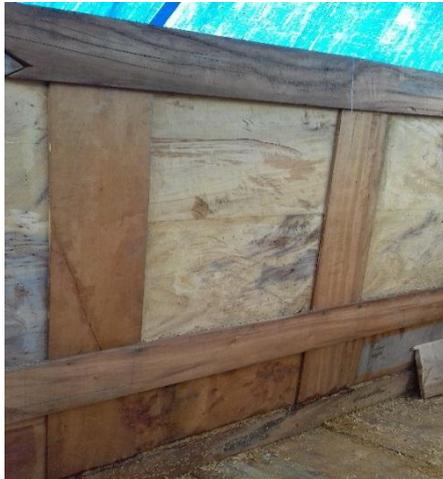
Figure 1. Wall installation (Rinding angin or Rimbang)
